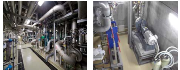
Fig. 2. Photograph of the cooling-water pump on the first floor and the SHARAQ water-cooling system.
