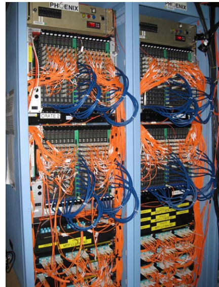
Fig. 1. The installed MuTRG-MRG and MuTRG-DCMIF boards.
