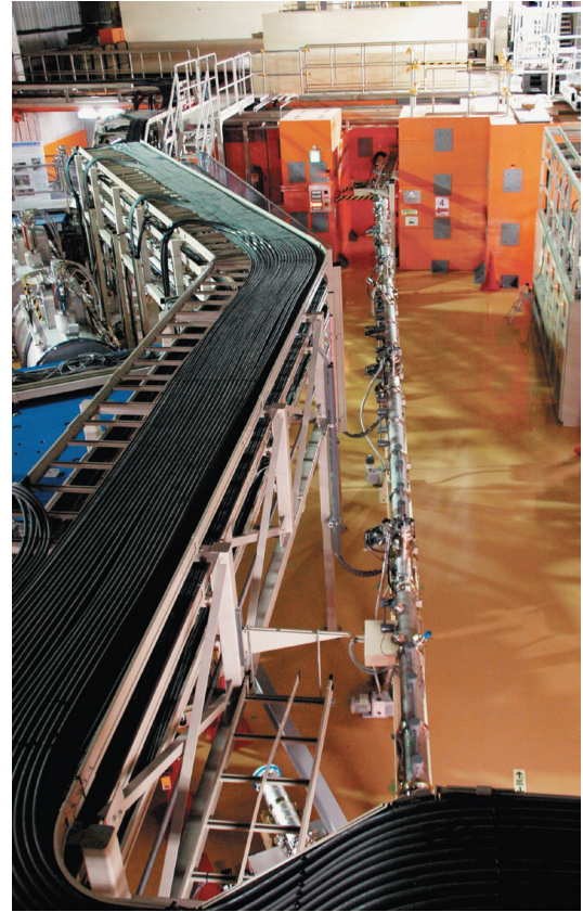
Fig. 1. Part of SLOWRI beam transport line, under installation.
