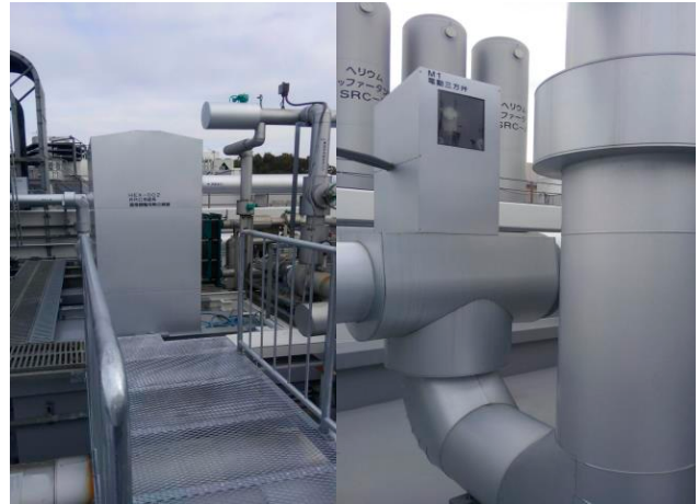
Photograph of the RRC Cooling capacity augment equipment
