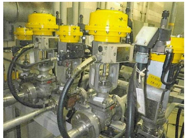
Fig. 2. Control valve unit in the RIBF compressor room.
