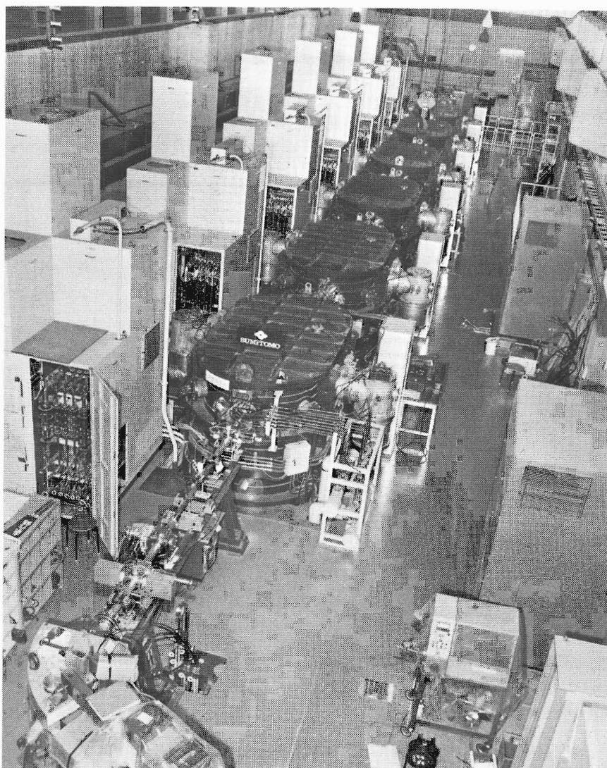
Fig. 1. The resonators and amplifiers in the accelerator vault, July 1979.
