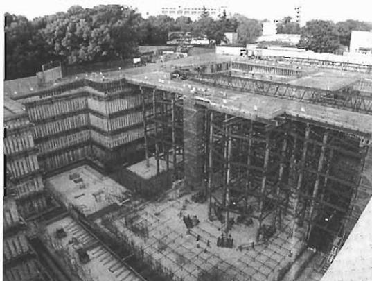
Fig. 2. Photograph of the SRC vault in April 2001. The bases for the sector magnets can be clearly seen.
