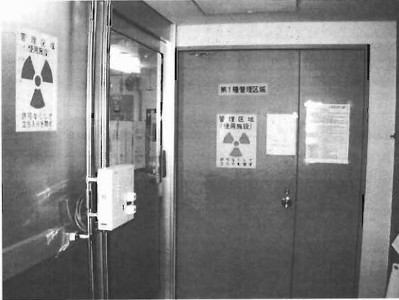
Fig. 3. The automatic door and the barcode reader in the RILAC contamination test room. The door on the left with a glass window is the automatic door, and the barcode reader is to the left of the door.
