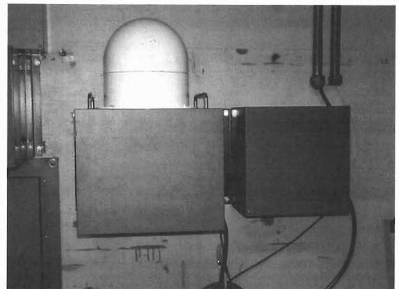
Fig. 2. The movable-head type radiation monitor in the 2nd basement corridor of the Nishina Building.
