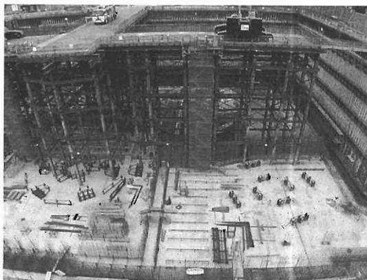
Fig. 1. Photograph of the SRC vault along with the IRC vault in April 2001. The bases for the sector magnets of both cyclotrons can be seen.
